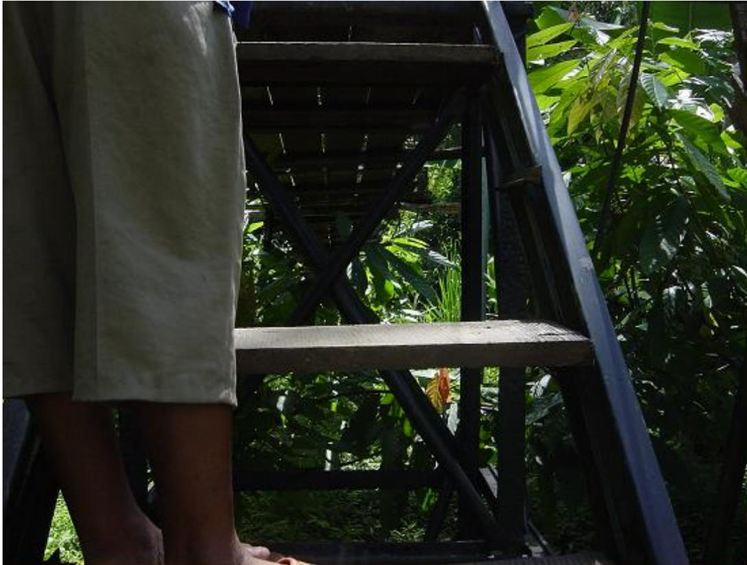
*One of the steps on the way up to the bridge has simply rotted out. Some of the boards on the bridge floor have broken. Cables are rusting out, and a few of them have been replaced. More work needs to be done to bring this bridge back to a safe condition.*
